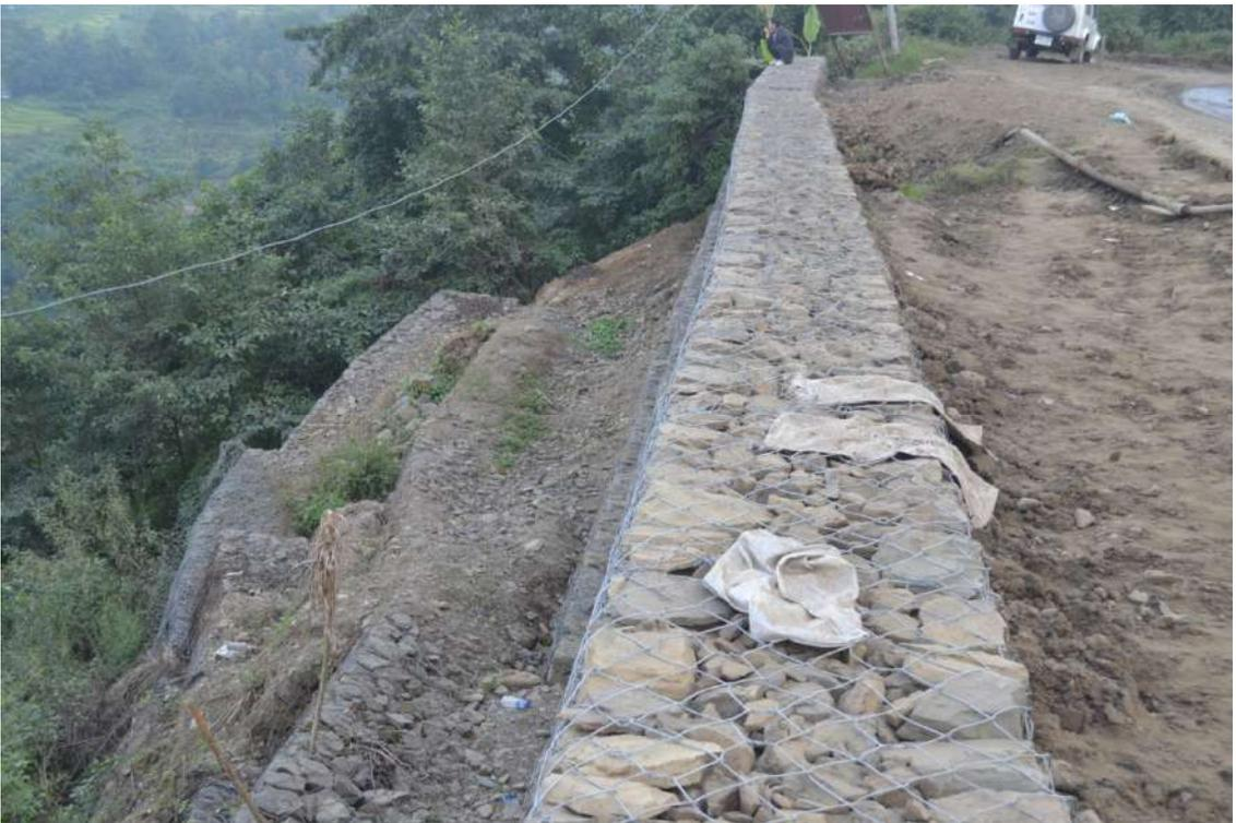
**Plate 7.1.a** Creeping indicated in man made structure
